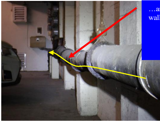
Some leaking joints are just packed with additional material
