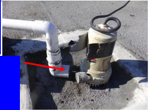
The roof has added drain area pumps where two did not respond, some have deteriorated roofing materials where water can enter...
