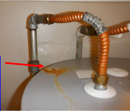
...the water heater has a leaking pipe fitting...
