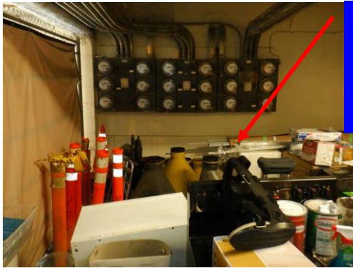
The SE-electrical service area lacks service clearance due to storage...
