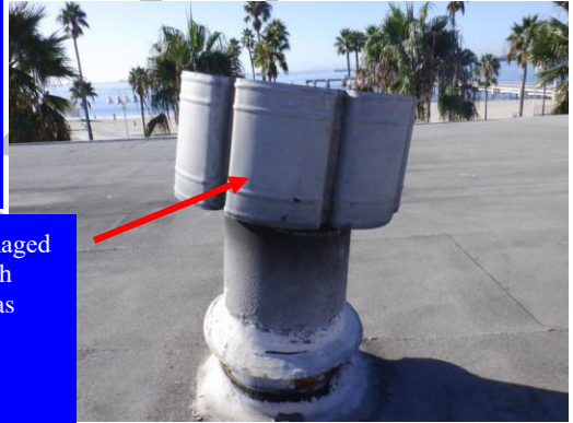
306A: The proper chimney cap is collapsing...
