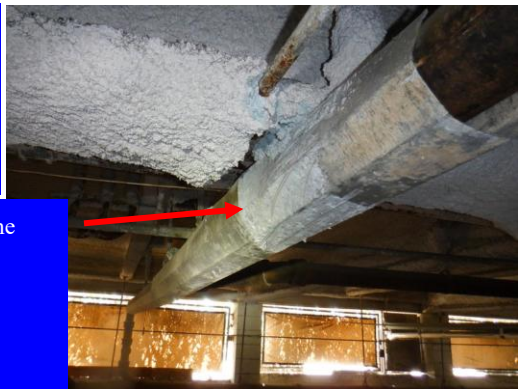
...a damaged waste pipe cap was noted near column #47...
