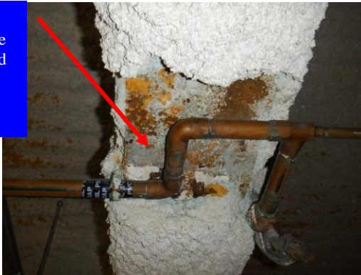
The garage support column adjacent to the pool equipment room required repairs following an auto impact
