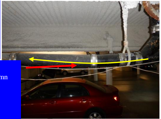
...and wrapping leaking waste pipes were conspicuous throughout the garage...
