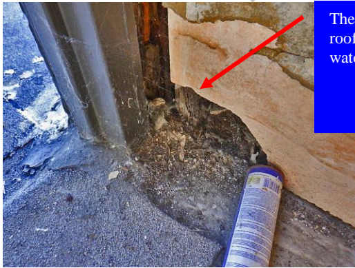
The terrace surface drains discharge against the building
