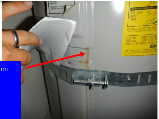
Unit #304: The water heater has corroded fittings...
