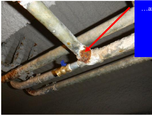
The waste piping in the garage has a number of leaks...
