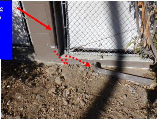
302...and one has a detached drain pipe
