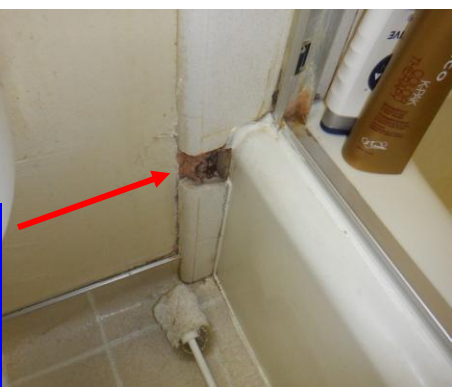
...the wall adjacent to the tub/shower is damaged...
