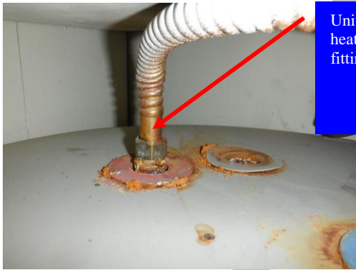
Unit #304: The water heater fittings are leaking
