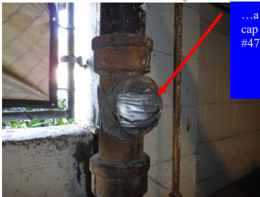
...again, shielding of the waste piping...
