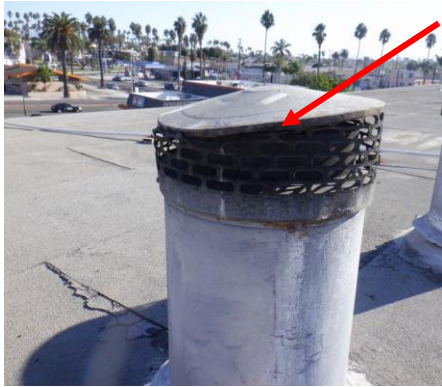
306A: The proper chimney cap is collapsing...
