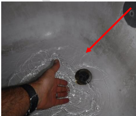
...the tub drain has backed-up...
