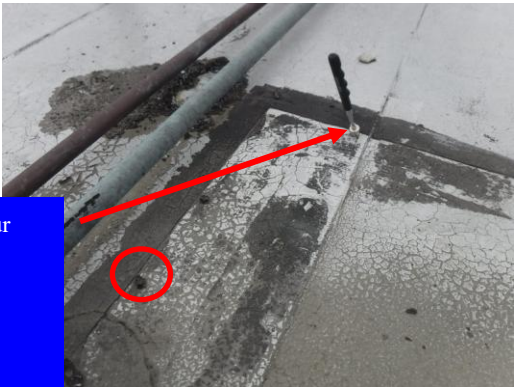
Other patched areas of the roof have 'popped' fasteners here demonstrated with a magnet...
