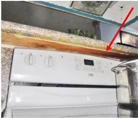
...the kitchen peninsula's combustible wood rough top hangs over the cooktop console and shows heat damage
