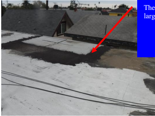
...lifting seams, cracked & crazed surface...
