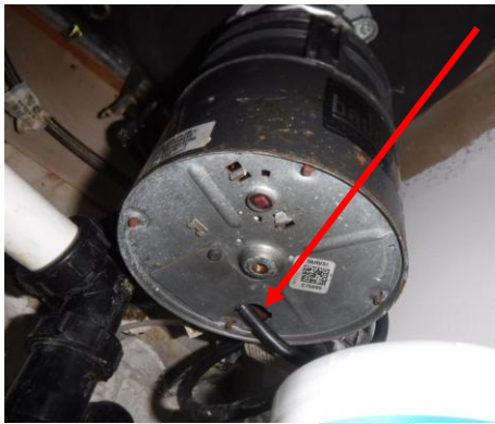
... the disposal unit power cord lacks a bushing
