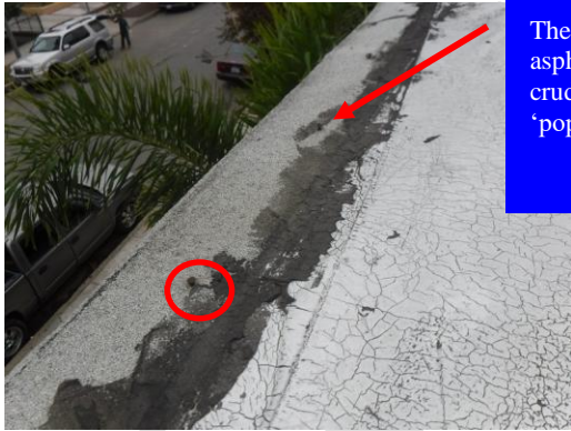
...and damage due to excessive over-hang
