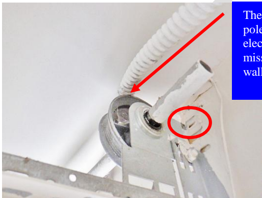
The garage attic fire separation wall is damaged
