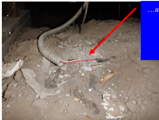
...and open electrical boxes were noted at the dining room crawl space...
