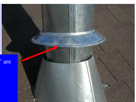
The water heater and forced air heater exhaust vent pipes are sealed to the flashing...
