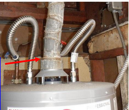
The water heater exhaust venting system has a reducer fitting and re-uses the corroded vent pipe that served the previous water heater
