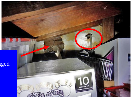
The vehicle door S-torsion pole drum is rolling against electrical conduit and missing lag screws at the wall mount
