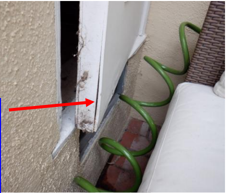
...the water heater closet door and casing are damaged...
