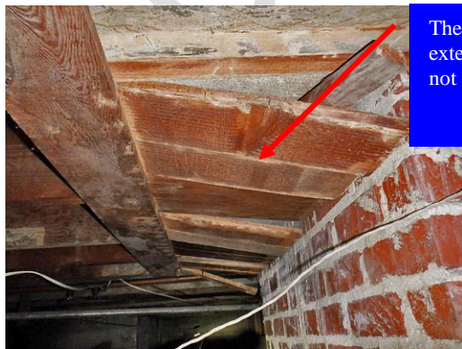
The kitchen crawl space has an added post with under-sized 'girder' when two posts are needed with a box girder as well as proper footings and framing hardware
