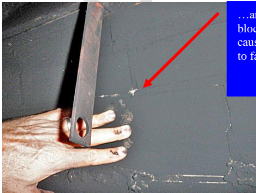
The full bath shower partition wall tile show water saturation
