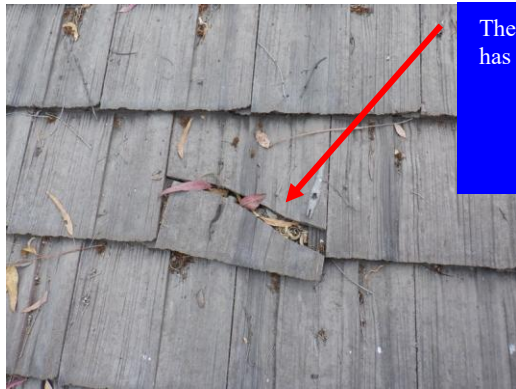
...and other tiles were noted to have developed cracks such as again at the garage E-slope...
