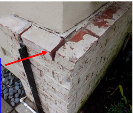
The exterior wall brick skirt has a few loose bricks...
