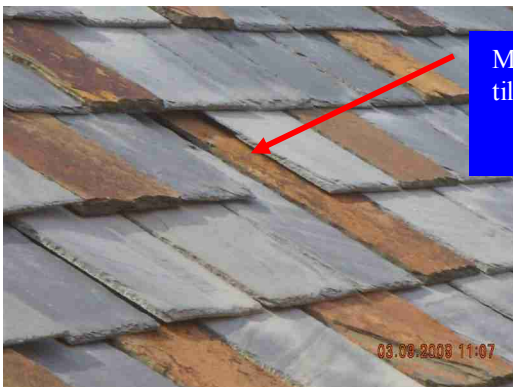
Missing/damaged slate roof tiles & exposed nails
