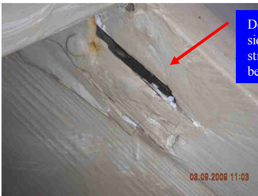
Stucco finish cracks
