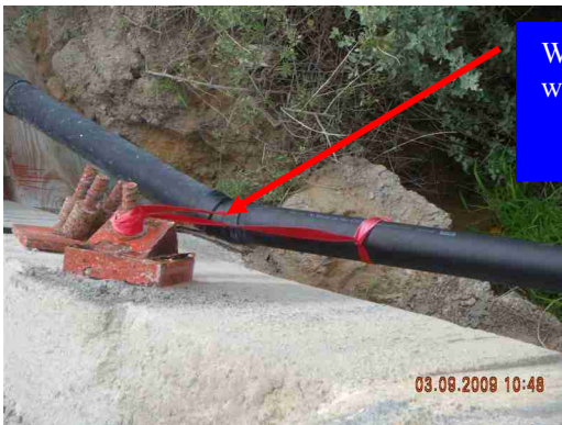
Loosening waste pipe connection at W slope
