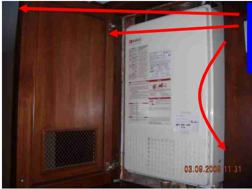
Tankless water heater in alcove without sufficient clearance from combustibles
